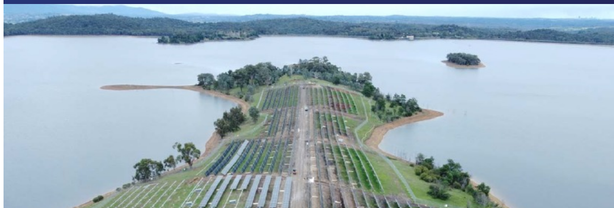
Beon constructed solar farm at Melbourne Water's Winneke Treatment Plant.
