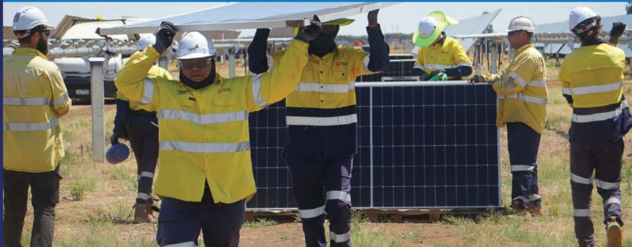
Participants in the Beon Aboriginal Training and Employment Program installing panels at the Avonlie Solar Farm.
