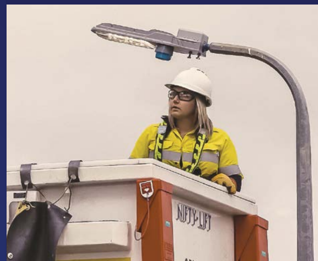
Teams have replaced over 20,000 streetlights in Geelong with energy efficient LED options to help reduce carbon emissions.
