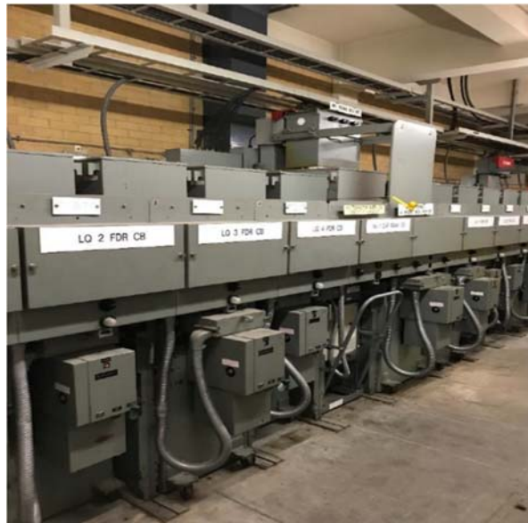
Existing Email HQ compound filled double bus switch board - Bus A shown
